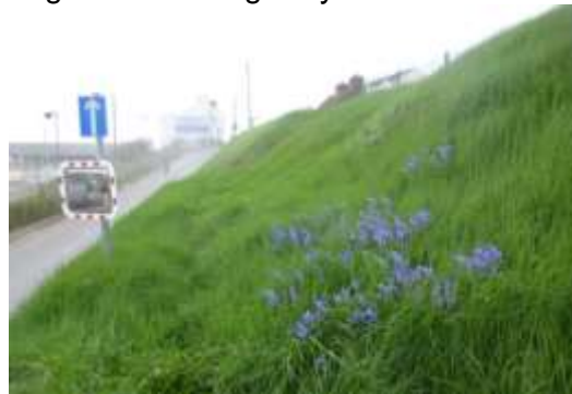
Basin Road North embankment
