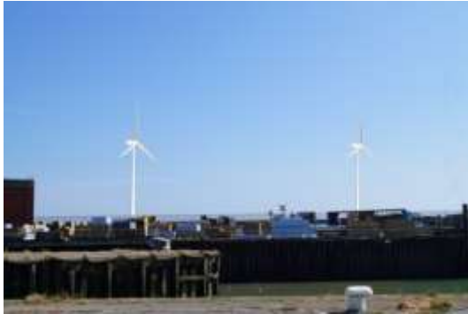
Wind turbines at Outer Layby
