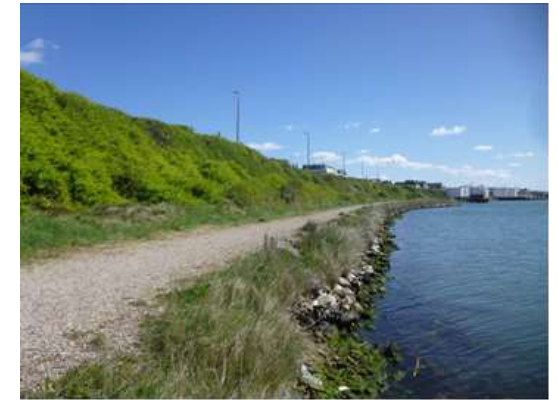
North Canal Bank
